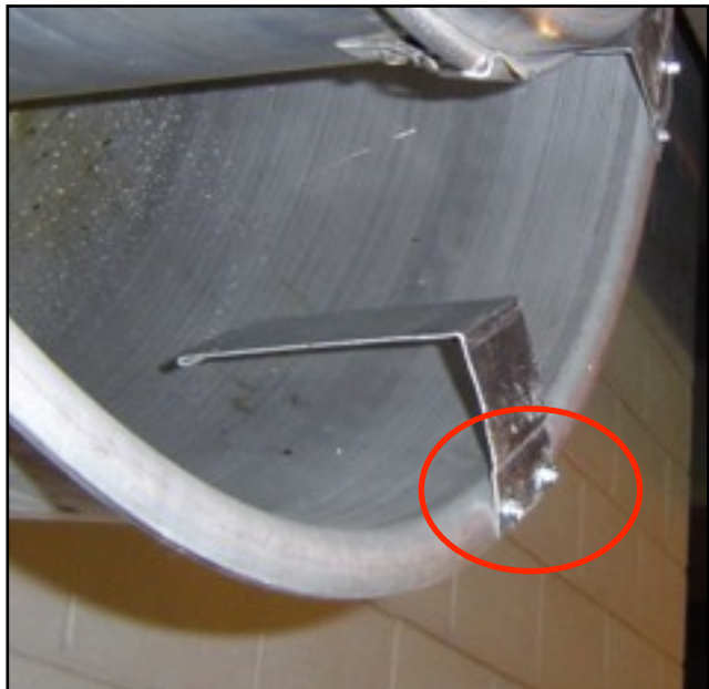
Pic #1 Installing Socket Brackets
