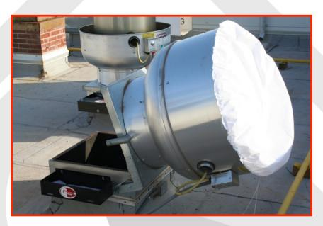
Spray wash caps play a vital role in controlling over spray when cleaning the under side of the exhaust fan. Over spraying equipment like AC coils, motors, light systems and property roofs can be extremely costly but easily avoided by utilizing this inexpensive solution. Your company will not only save time and money but will also help ensure the environment will stay grease free by keeping greasy wash water contained.
