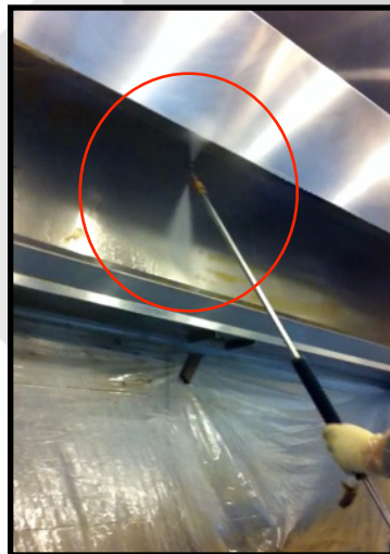
Spraying Top Track
